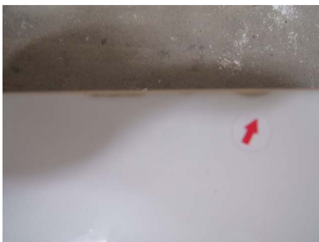
lost glaze on top edge of tank
